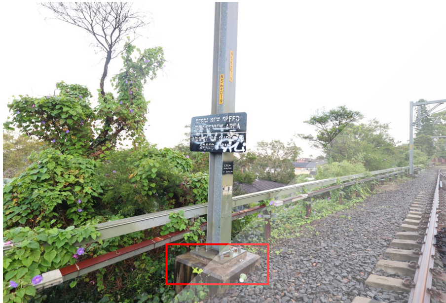
General view of the overhead structure NS 6+019 on the south side of the railway. Showing slight chipping on concrete footing.
