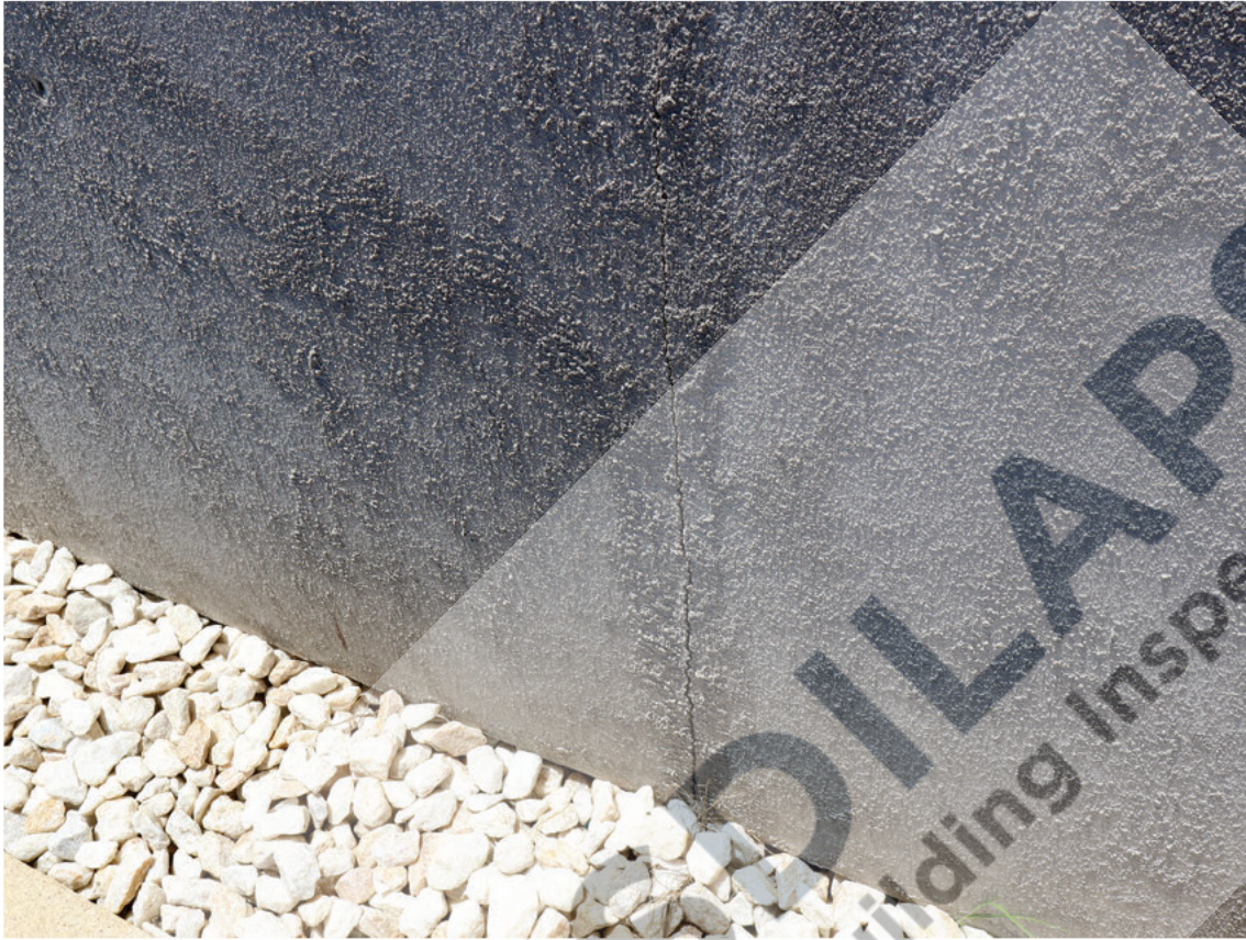
Picture 4 – Vertical alignment of crack- Figure No 257 from the Post report
