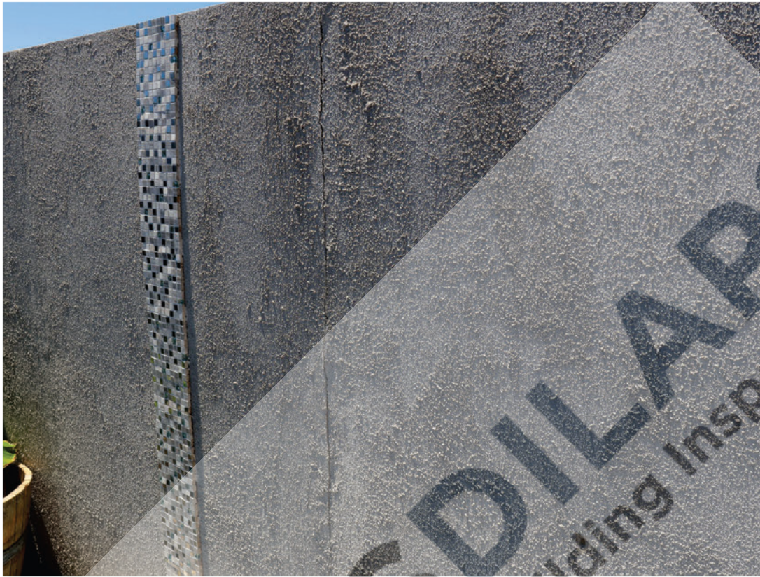
Picture 5 – Vertical alignment of crack- Figure No 258 from the Post report
