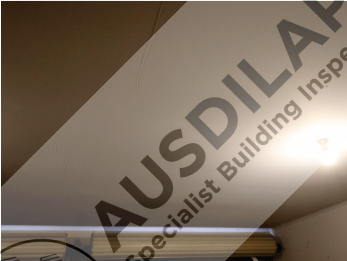
Picture 1 - Bubbling paint in the ceiling in the garage- Figure 113
