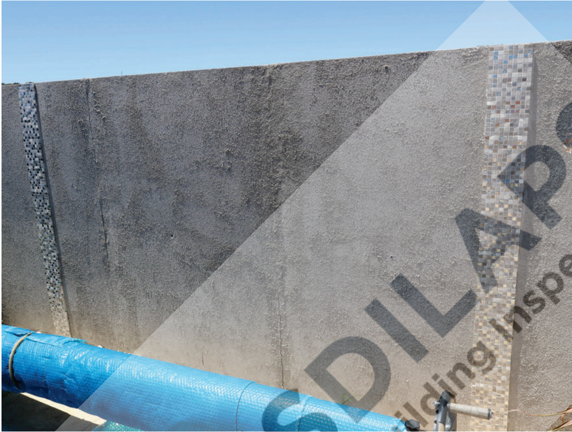
Picture 3 – Vertical alignment of crack- Figure No 256 from the Post report
