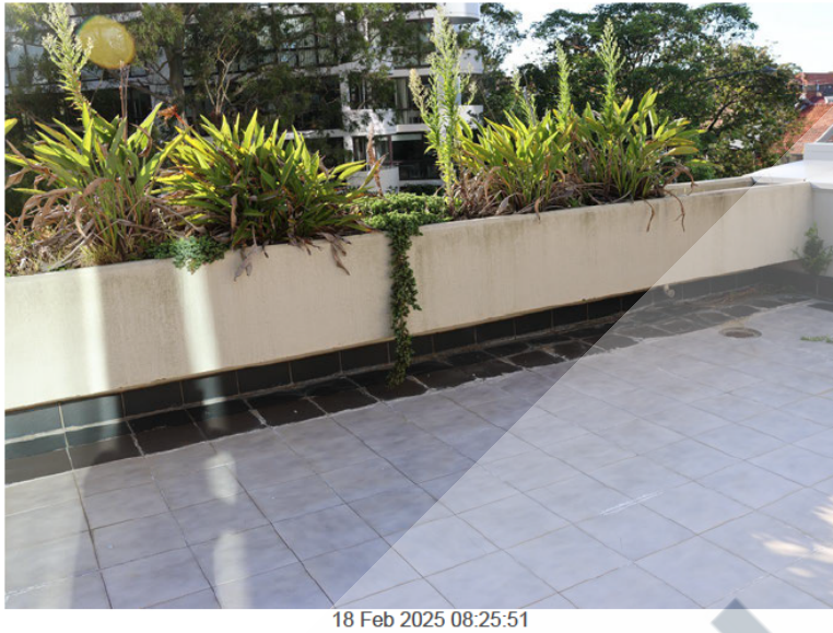
East retaining wall on the level 3 balcony, south side.
