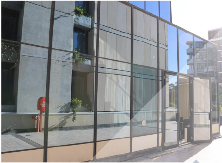
North wall on the level 3 balcony.
