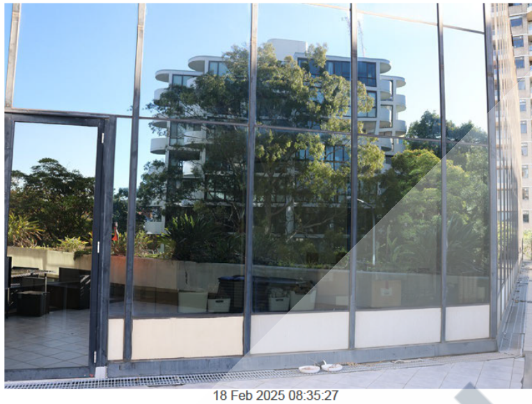
North wall on the level 3 balcony, east side.
