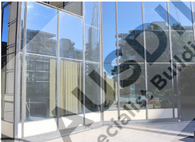
North wall on the level 3 balcony, east side.
