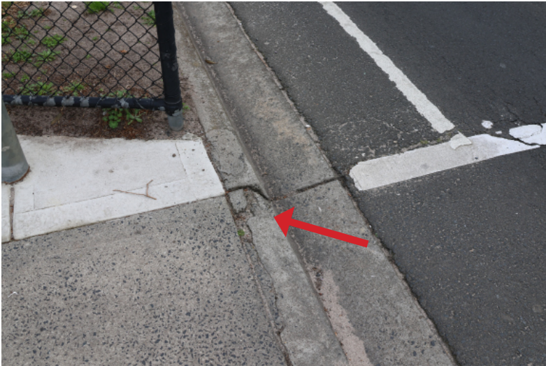
Figure: 0055 Chipping in the kerb on Booran Road.
