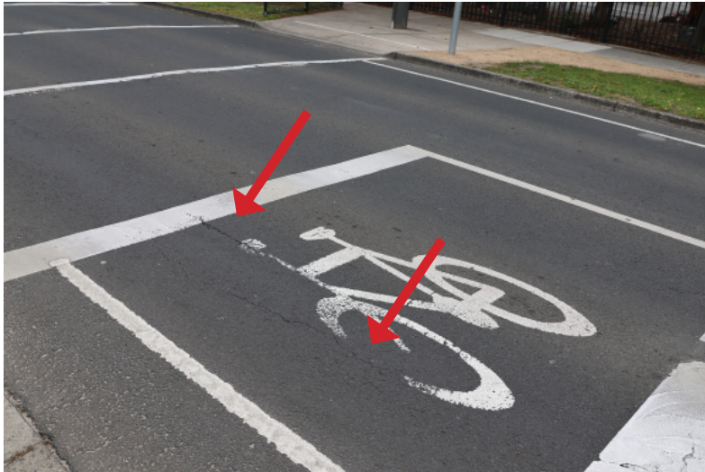
Figure: 0043 Slight cracking in the roadway on Booran Road.
