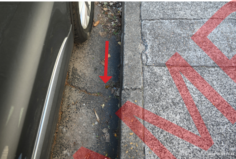
Figure: 0029 Cracking in the kerb and gutter.
