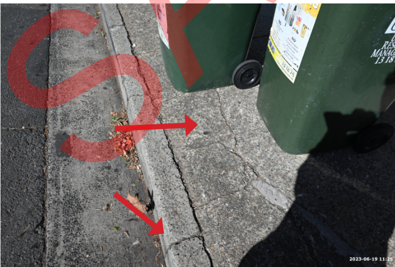
Figure: 0036 Cracking in the footpath and kerb.
