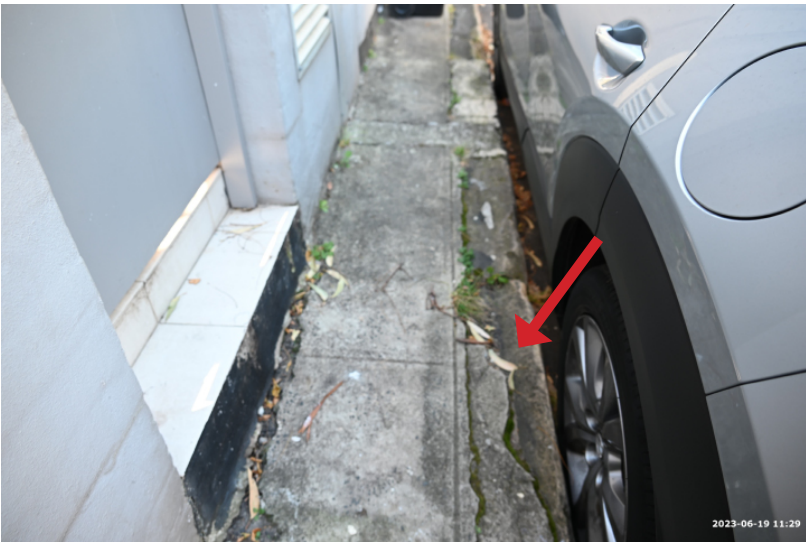
Figure: 0064 Damage in the kerb in the laneway.
