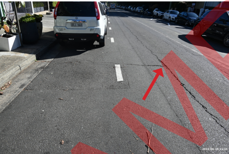
Figure: 0041 General view of the roadway. Showing cracking.
