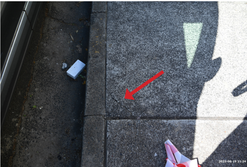
Figure: 0028 Cracking in the footpath.
